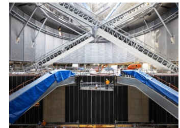
C Hoisting the escalator onto its supports
