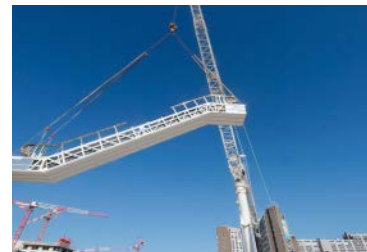
B Moving the escalator into the building
