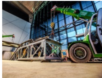
A Transportation to the installation site using special forklift trucks
