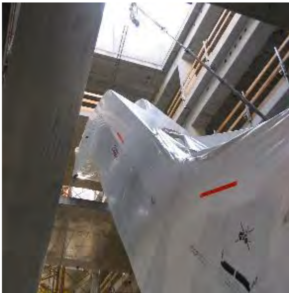
Installation in one complete section by crane
